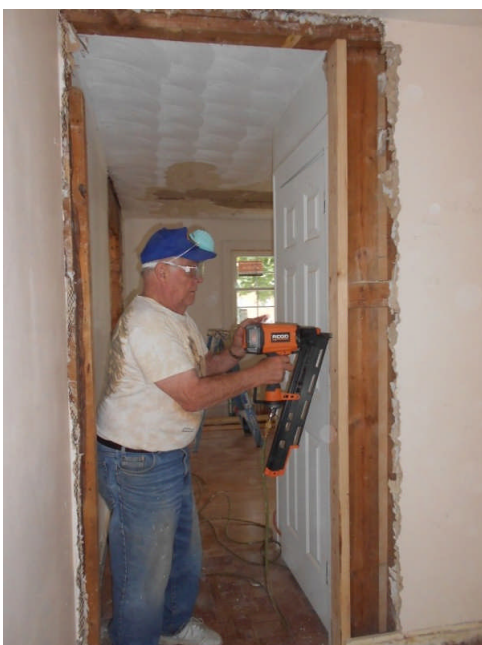
PDG Lion Jerry DeGraff working the nail gun while installing new headers for the wider doorways.
