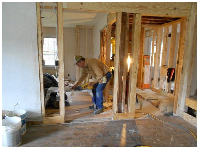
PDG Lion Jerry DeGraff working the nail gun while installing new headers for the wider doorways.
